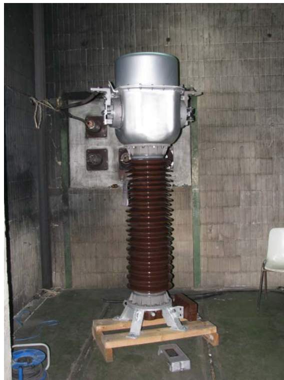
Short-circuit test lay-out.
