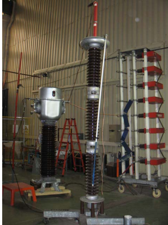
Lightning impulse test lay-out.
